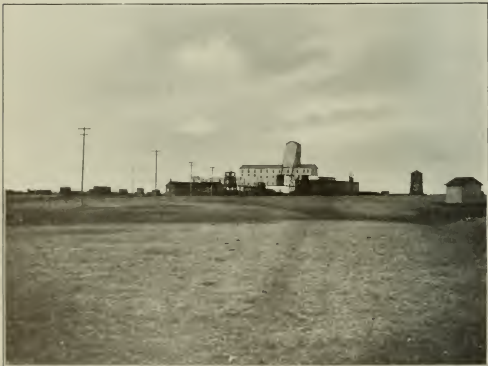
The Lethbridge Coal Co. (No. 6), Lethbridge, Alta.
